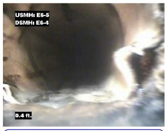
**Distance:** 0.4 ft. **Grade:** 3 **Condition:** Lining Failure Defective End
