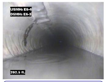
**Distance**: 202.5 ft. **Grade**: 3 **Condition**: Lining Failure Delaminating
