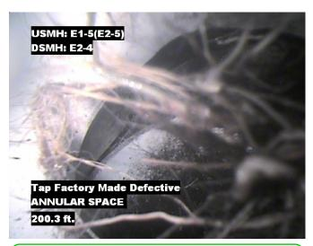
**Distance**: 200.3 ft. **Grade**: 2 **Condition**: Tap Factory Made Defective
