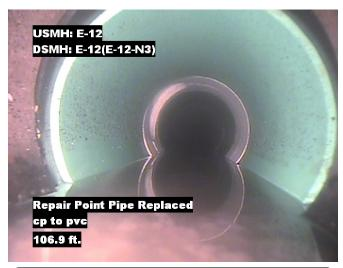
**Distance**: 106.9 ft. **Grade**: 0 **Condition**: Repair Point Pipe Replaced
