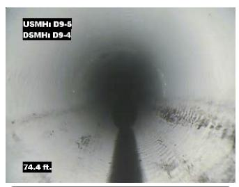
**Distance**: 74.4 ft. **Grade**: 0 **Condition**: Repair Point Pipe Replaced
