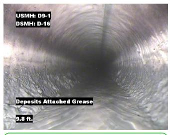
**Distance**: 9.8 ft. **Grade**: 2 **Condition**: Deposits Attached Grease
