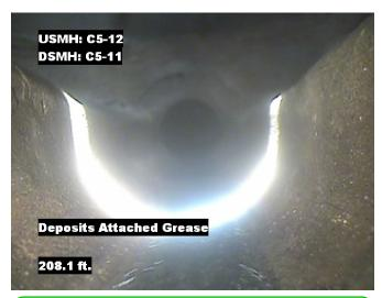
**Distance**: 208.1 ft. **Grade**: 2 **Condition**: Deposits Attached Grease
