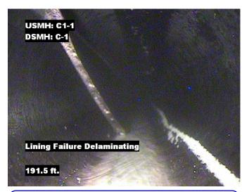
**Distance**: 191.5 ft. **Grade**: 3 **Condition**: Lining Failure Delaminating
