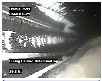
Distance: 29.8 ft. Grade: Condition: Lining Failure Delaminating
