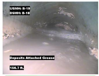
**Distance:** 156.7 ft. **Grade:** 2 **Condition:** Deposits Attached Grease
