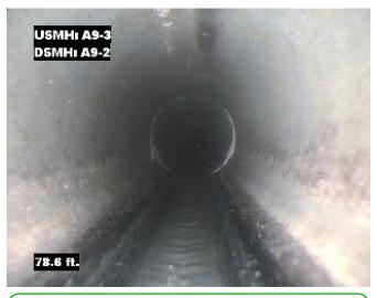
**Distance**: 78.6 ft. **Grade**: 2 **Condition**: Deposits Attached Grease
