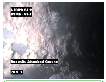
**Distance**: 78.9 ft. **Grade**: 2 **Condition**: Deposits Attached Grease
