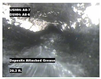
**Distance**: 20.2 ft. **Grade**: 2 **Condition**: Deposits Attached Grease
