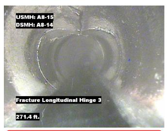
**Distance**: 271.4 ft. **Grade**: 5 **Condition**: Fracture Longitudinal Hinge 3
