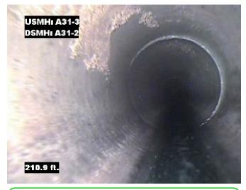
**Distance**: 210.8 ft. **Grade**: 2 **Condition**: Deposits Attached Grease
