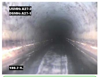
**Distance**: 190.3 ft. **Grade**: 2 **Condition**: Deposits Attached Grease
