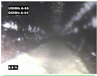
Distance:6.5 ft.Grade:2Condition:Deposits Attached Grease
