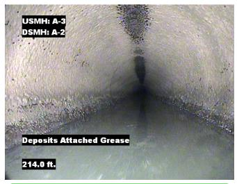
Distance: 214.0 ft. Grade: Condition: **Deposits Attached Grease**
