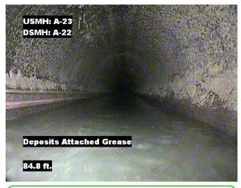
Distance:84.8 ft.Grade:2Condition:Deposits Attached Grease
