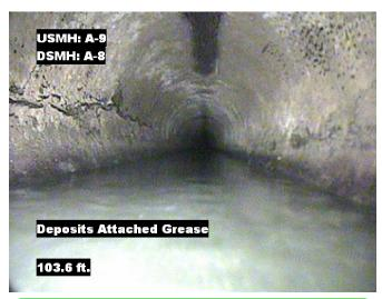
**Distance**: 103.6 ft. **Grade**: 2 **Condition**: Deposits Attached Grease
